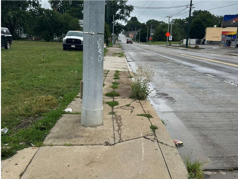
Figure 15. A pole blocks wheelchair access near Wyoming Street
