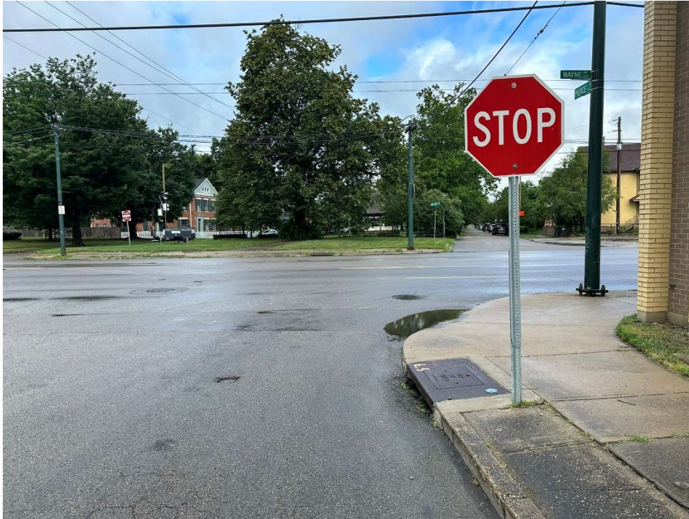
Figure 13. Limited sight distance when traveling westbound on Pierce Street
