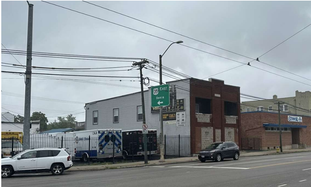
Figure 6. Visual and physical clutter: utilities and US 35 signage
